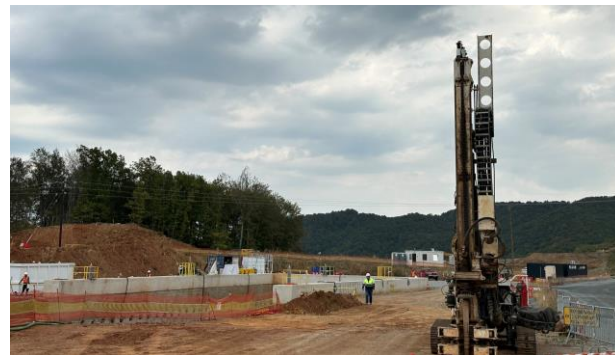
Primary crusher foundation
